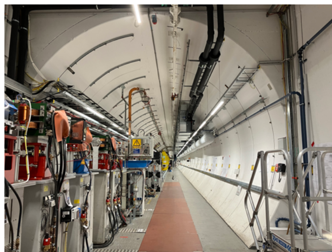
Fig. 2: View into the filled FLASH1 tunnel close to the shutdown end (photo: K. Honkavaara, taken on July 31, 2025). In the background one sees some of the yellow frames of the new Apple III undulators and at the top right the new air-conditioning.
