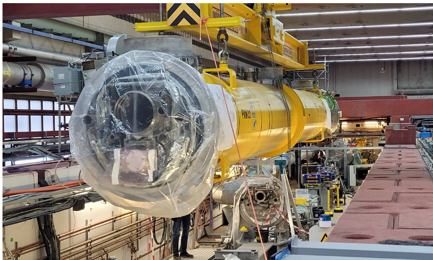
New accelerating module being hoisted to its destination in the accelerator tunnel. Compared to the original modules the new ones support an increased accelerating gradient and thus will allow an by 100 MeV increased energy gain.
