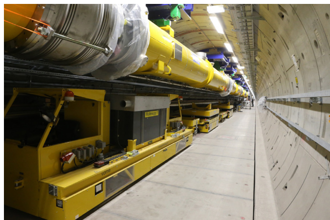
The first accelerator modules installed in the underground tunnel of European XFEL.
