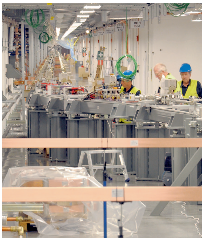
The 350 m long linac tunnel where installation of the 3 GeV linac is now completed (seen from the gun hall with the first bunch compressor).
