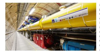
Free-electron lasers are powered by high performance electron accelerators and are usually built in dedicated tunnels. The European XFEL, for example, is located underground where a 1.7 km long accelerator brings electrons to the high energies necessary for X-ray generation.
