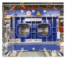
An APPLE-X undulator installed in the European XFEL photon tunnel
